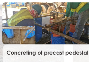
Checking of actual top and bottom covering
