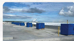
Installation of ACCU units at Roof Deck
