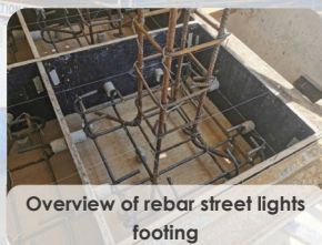
Checking of actual form dimension (Length x Width)
