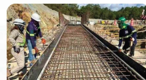
Concrete Spillway inspection - Width
