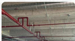
Installation of sprinkler branches and cross main pipe
