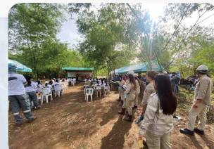
Laying of concrete samples for compressive test
