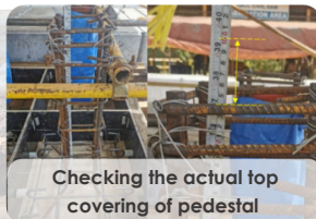
Overview of rebar street lights footing
