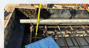
Concrete Spillway inspection - Depth
