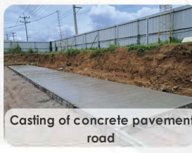
Slab-on-grade concreting works for Production Area
