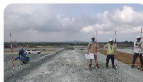
Dam Crest Internal Inspection - Overview
